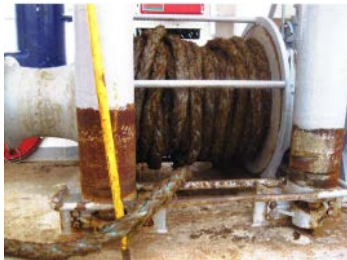
Front view showing mooring line travel to the winch and the crow bar position.
